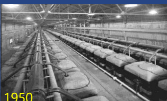
Hundreds of electrolytic cells, in row after row, work 24 hours a day at Hooker Electro-chemical producing the basic ingredients of all Hooker Chemicals. In each of the Hooker cells, under the action of direct electric current, salt and water are broken down into a constant flow of caustic soda, chlorine, and hydrogen.
